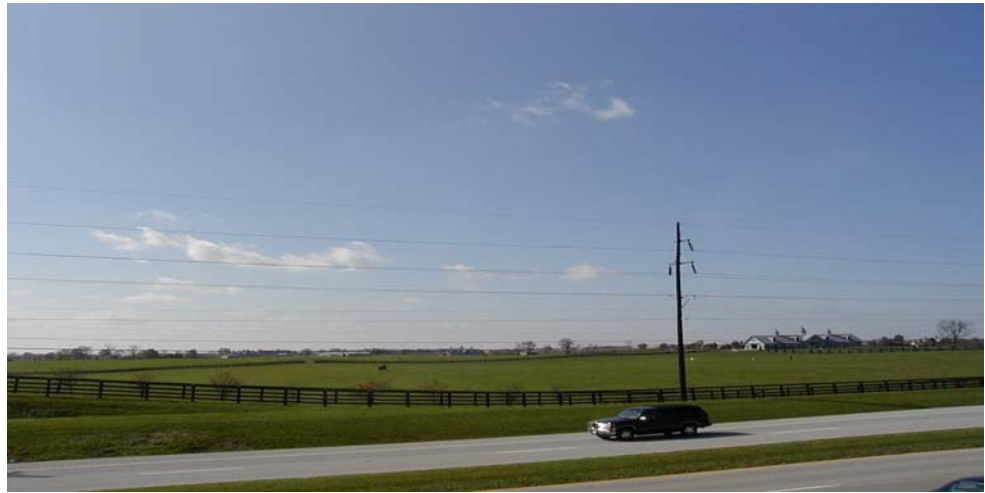
Example of a Viewshed – Looking southwest from US 60
